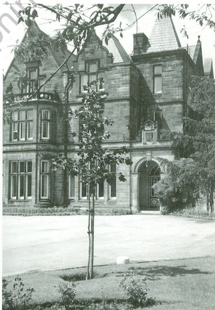
Front of School in 1993, featuring the canadian maple planted in 1990 by Richmal Ashbee, niece of Richmal Crompton.
